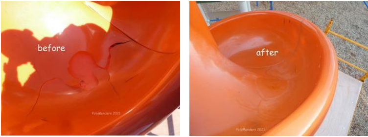
Slide repair at MLK Park
