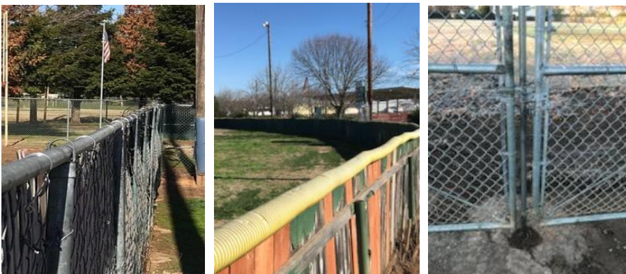
Fence line and gate repairs at Nolan Ball Fields
